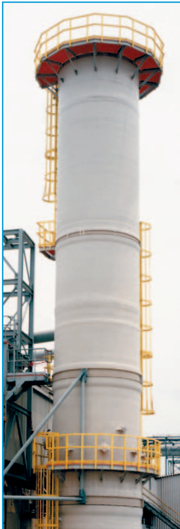
Chlorination tower has four caged ladders, each 30 ft. long.
