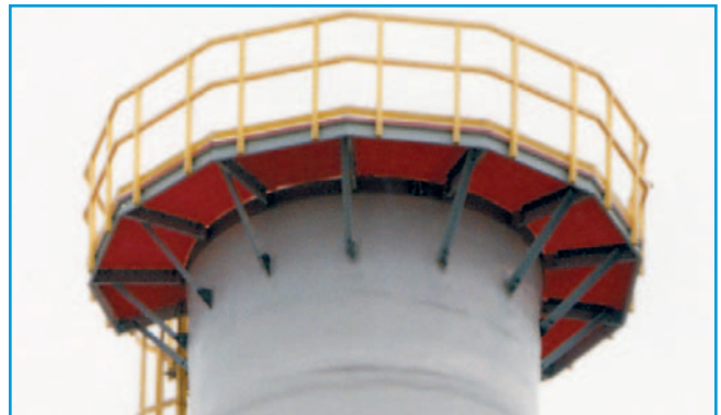
One of several perimeter platforms installed at various elevations.
