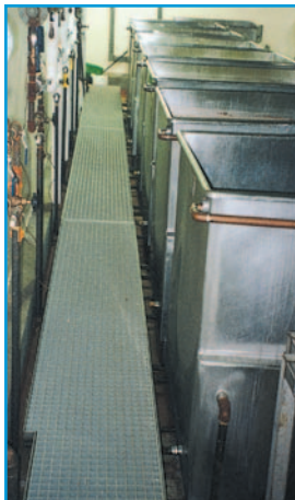
A GatorGrate Walkway runs the length of the cooking area.
